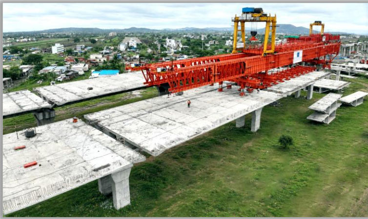
Pune Ring Road Project
