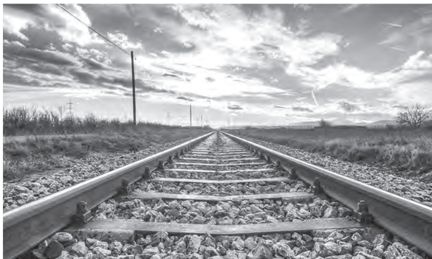
Trace construction at Eastern Dedicated Freight Corridor
